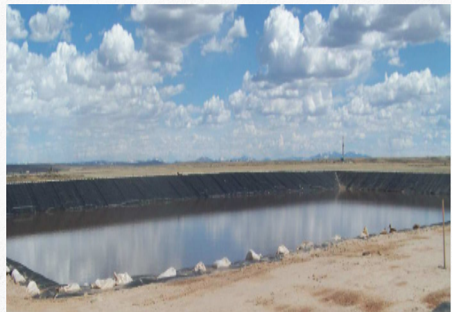
Figure 6: HDPE-Lined Water Disposal Pit
