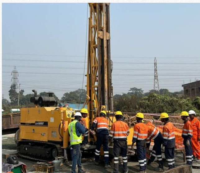
Figure 4: Drilling operation in Jharia CBM Block-I, CIL
